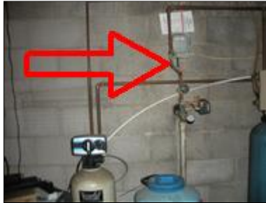
Main Water Shut-off
